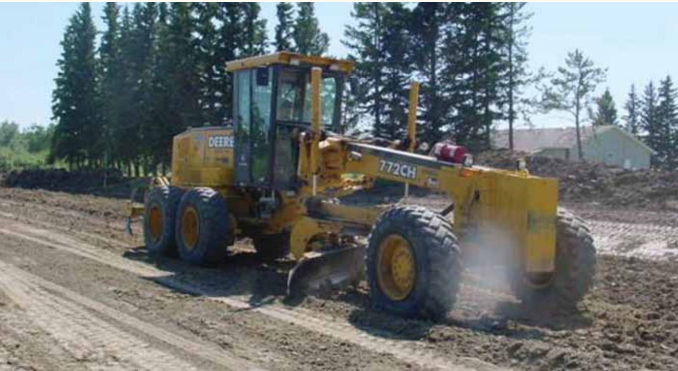
Preparing the ground for road construction
